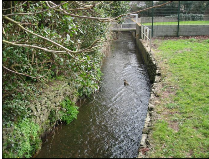
Plate 7: ICA Bridge on Ballybrack Stream eastern elevation
