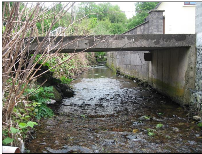
Plate 9: Middle Ravensdale Bridge on Ballybrack Stream, southern elevation
