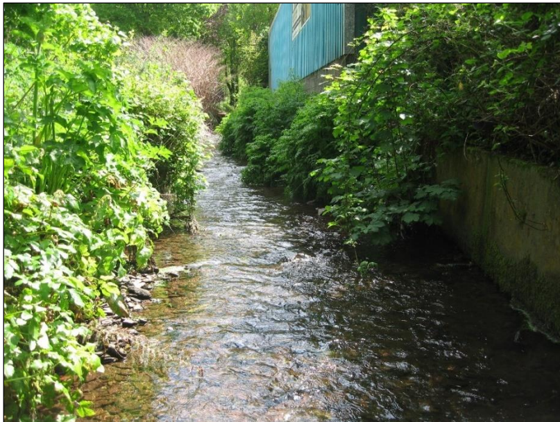
Plate 13.6: Concrete western bank of the Ballybrack Stream in Douglas Community Park, looking south
