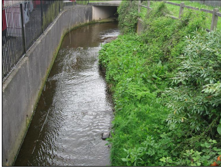
Plate 18: Tramore River emerging from culvert under Togher Road behind Greenwood Estate, looking west
