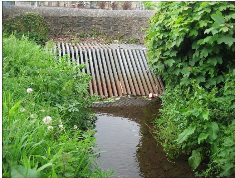
Plate 13.23: Tramore River entering culvert running under Togher Roundabout
