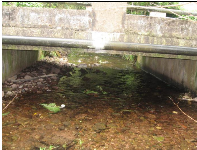
Plate 8: Lower Ravensdale Bridge on Ballybrack Stream, southern elevation
