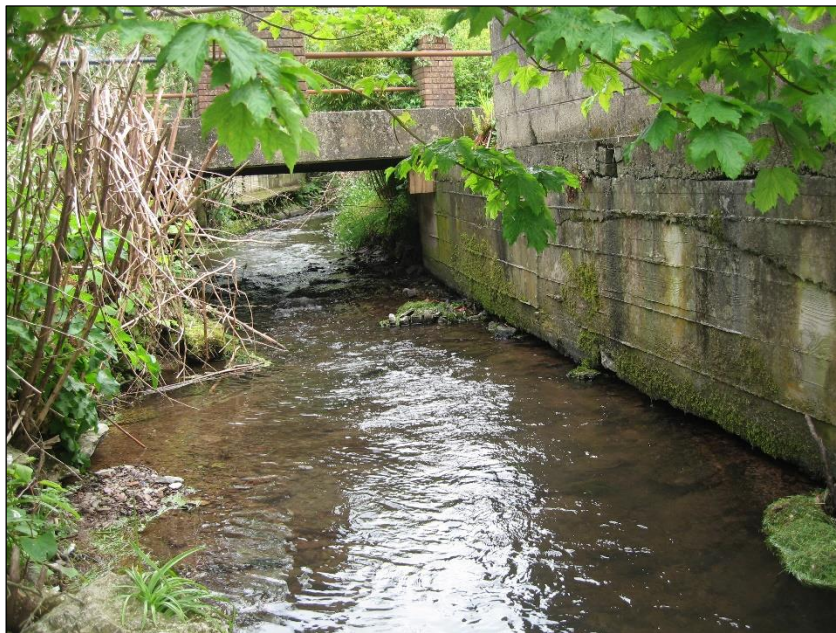
Plate 13.14: Ballybrack Stream in Ravensdale showing Upper Ravensdale Bridge, looking south
